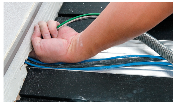
Run AC conduit through wall cutout
